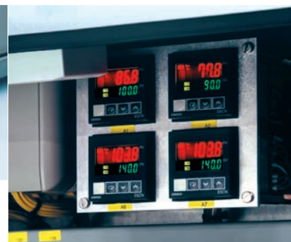
Omron's E5CN temperature controllers are used in Repak's machine control panels to control the heating.
